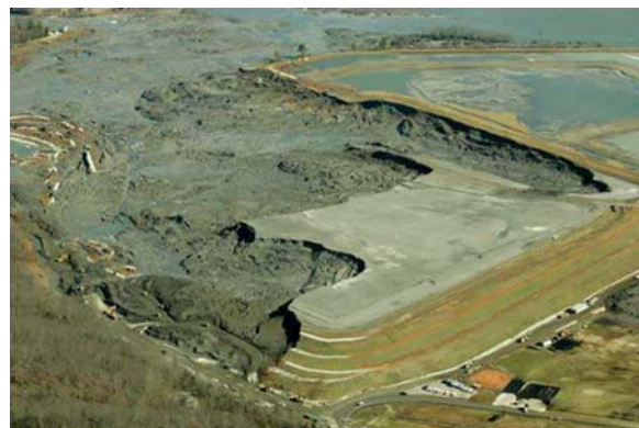
Figure 3. A coal ash slurry dump near the Kingston Fossil Plant in Harriman, Tennessee. Coal ash is composed primarily of oxides of silicon, aluminum, iron, calcium, magnesium, titanium, sodium, potassium, arsenic, mercury, and sulfur plus small quantities of uranium and thorium. Some of the uranium is U235, a fissile radioactive material together with thorium. Fly ash is primarily composed of non-combustible silicon compounds (glass) melted during combustion. Tiny glass spheres form the bulk of the fly ash. Stored coal ash slurries eventually threaten water supplies, human health, and local ecosystems. Photo: Wade Payne/Greenpeace, via Associated Press.
